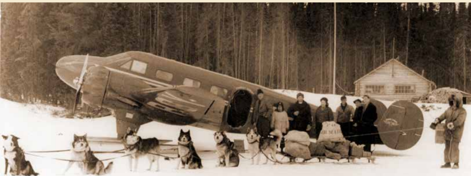
The first production Model 18A (S18A when equipped with floats) was purchased by Starratt Airways, located in Hudson, Ontario, Canada. It operated on skis as well as floats and landing gear, and was flown extensively in the Canadian bush country. The airplane was powered by two Wright R-760 radial engines, each rated at 320 hp. (WICHITA STATE UNIVERSITY
