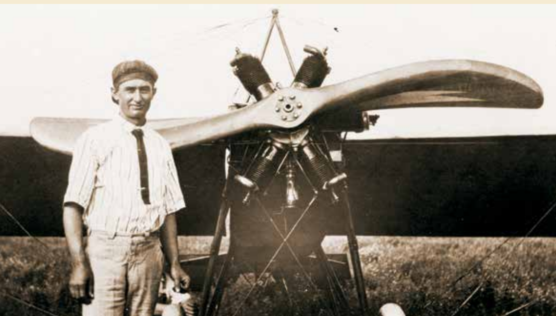
Clyde Cessna posed for the camera with his latest design he called The Comet . Built in 1917, the Anzani-powered monoplane featured a cockpit in front of the pilot that could accommodate a passenger, albeit a small one.
